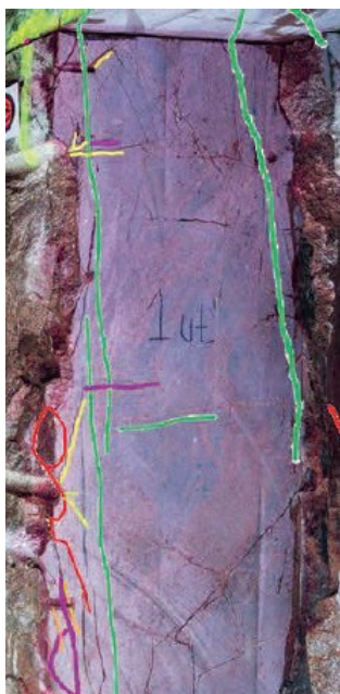
(a) Blast-induced cracks, field investigation
