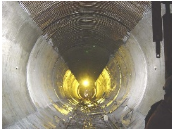
Figure 6: Headrace Tunnel with reinforced concrete
