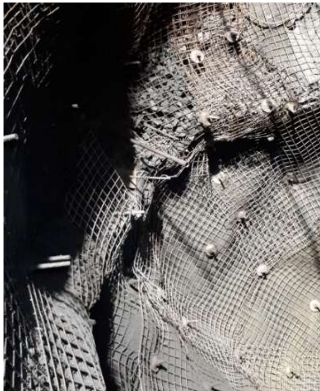
Figure 7. LKAB Malmberget, example area of difficult ground conditions
