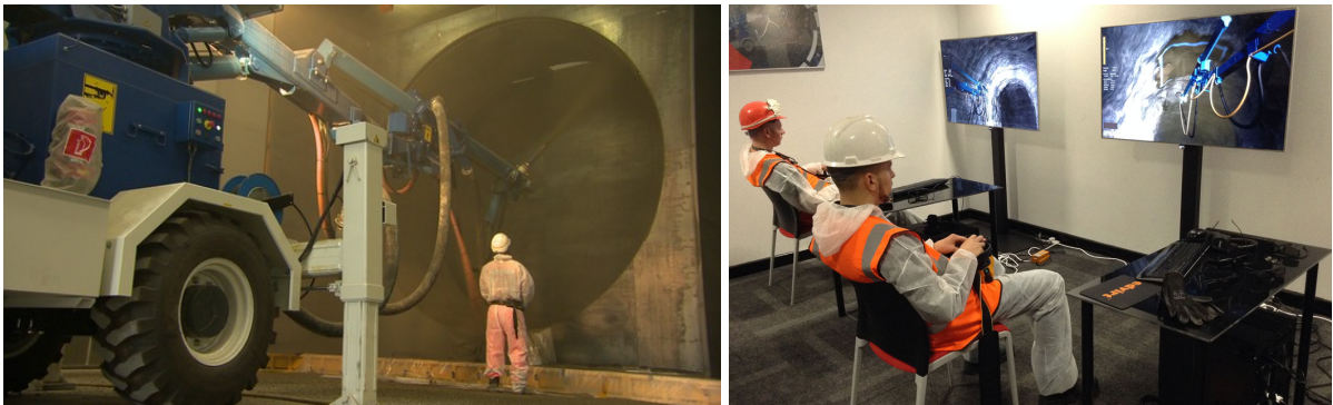
Photo 3: Training spraying in mandrels at TUCA. (Source: Ck-tech Ltd)
